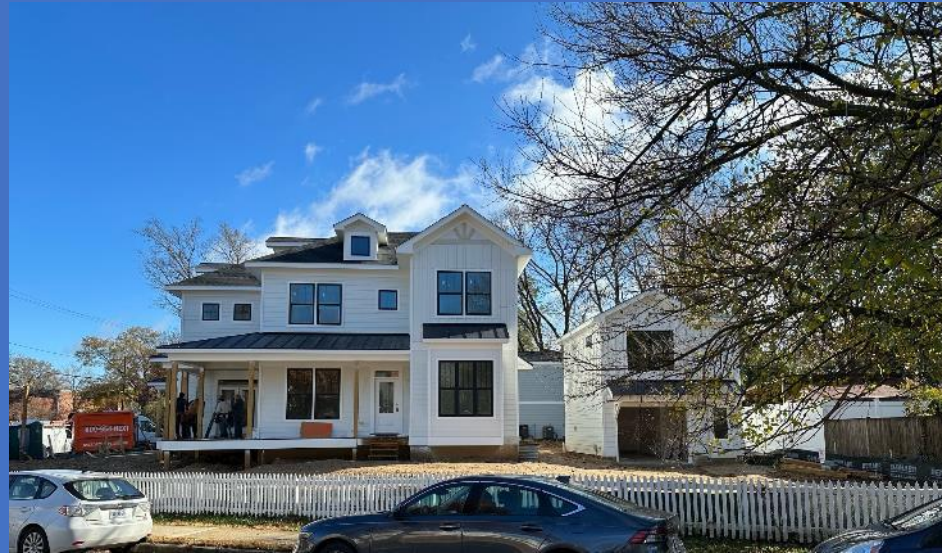
View facing Commonwealth
